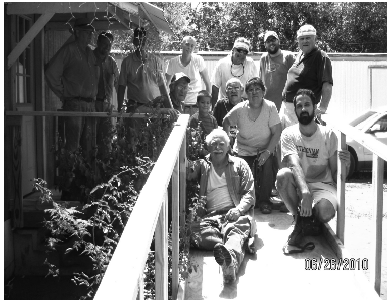
Workers and the Juarez family gather for a picture on the just-completed wheelchair ramp.
